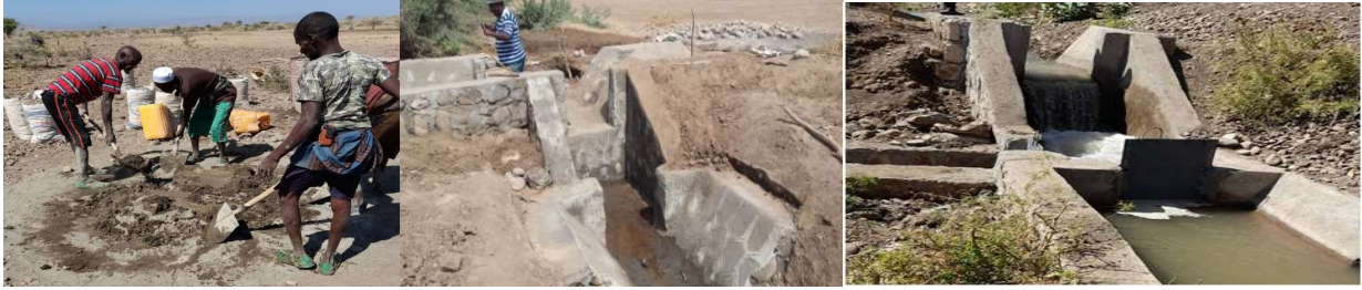
Figure 11: Drop structure constructed on the main canal
