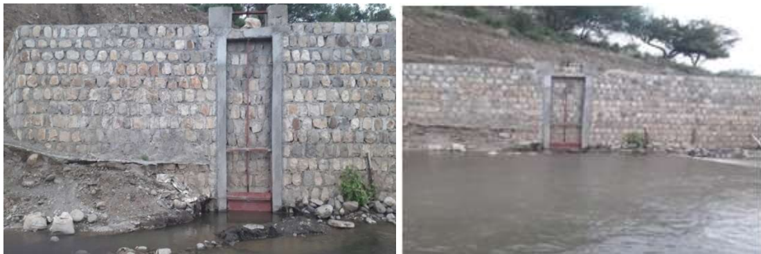
Figure 6: Main canal gate installed
