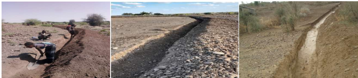
Fig 25: Cut off drain excavated
