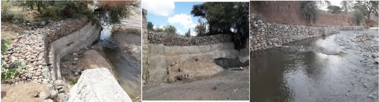
Figure 7: River protection work
