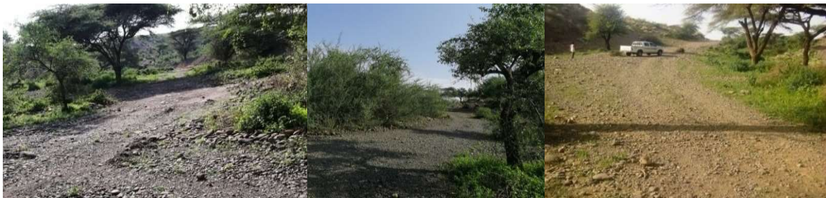
Figure 2: Road constructed and cleared
