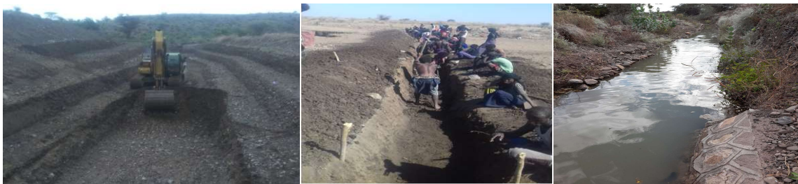
Figure 8: Main canal excavated by labour & machine
