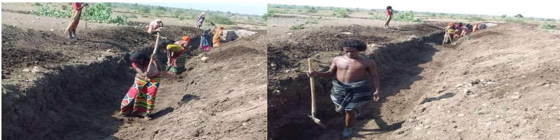
Fig 15: Secondary canal excavation by CFW participants
