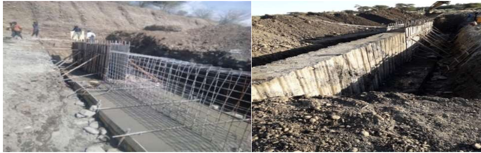
Figure 3: Concrete cut off wall constructed
