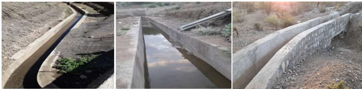
Figure 10: Lined canal constructed
