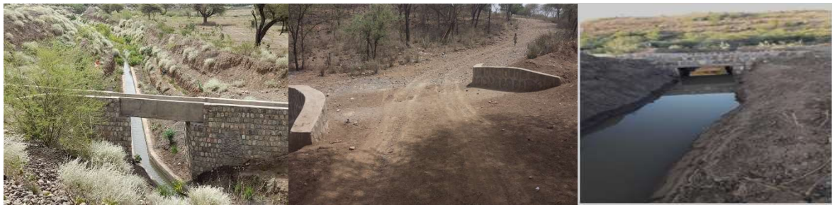
Figure 12: Road & drainage culverts constructed on the main canal
