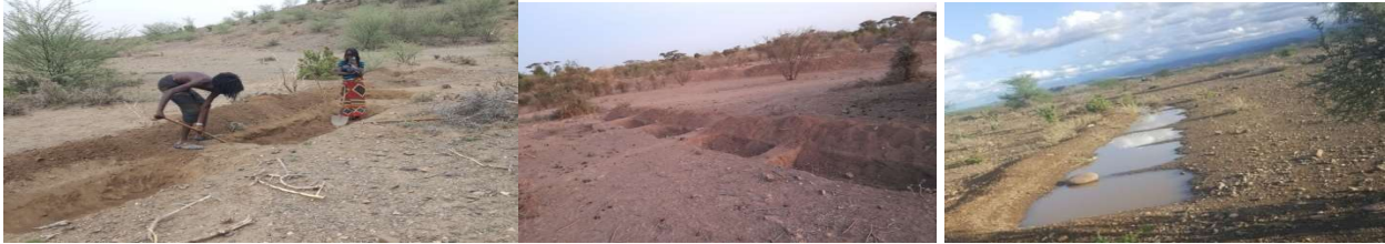
Figure 23: Soil bunds excavated
