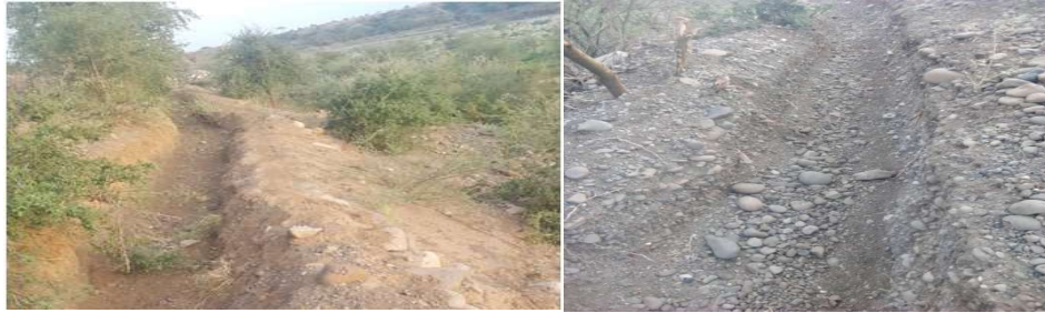
Fig 9: Drainage canal excavated
