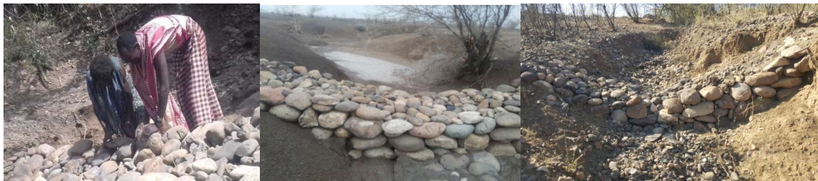
Figure 24: Stone check dams constructed
