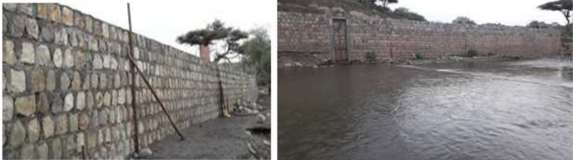
Figure 5: Retaining wall constructed
