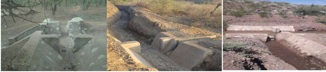
Figure 13: Division box constructed
