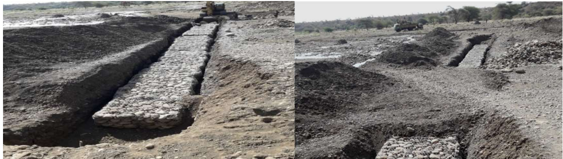
Figure 4: Gabion cut off wall constructed
